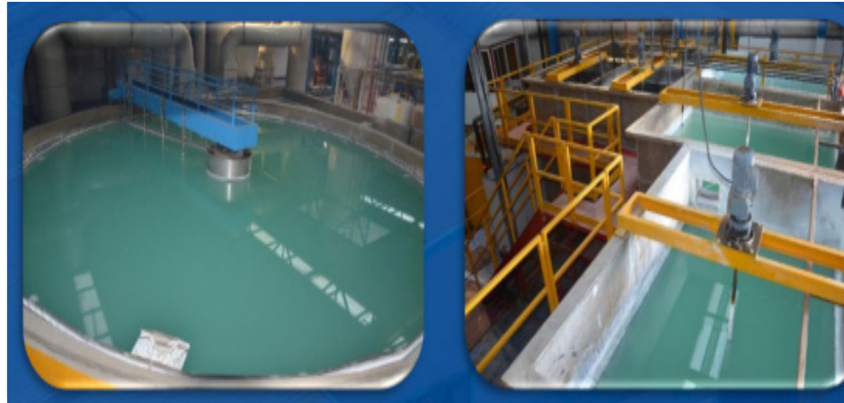
Esenyurt-Water Treatment Plant
