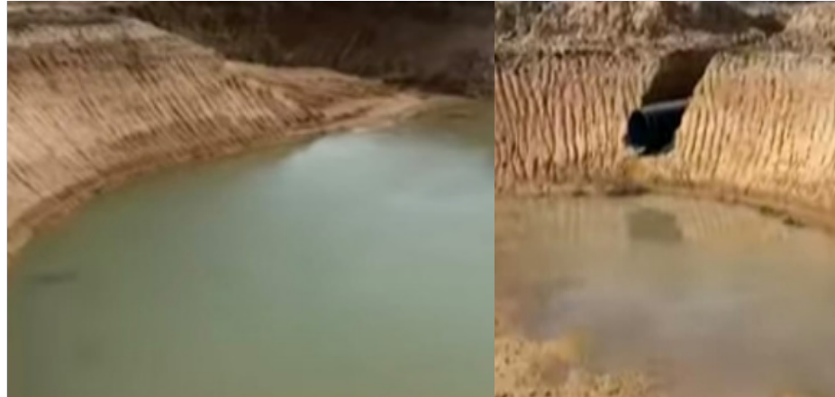
Kirklareli Water Storage Pool
