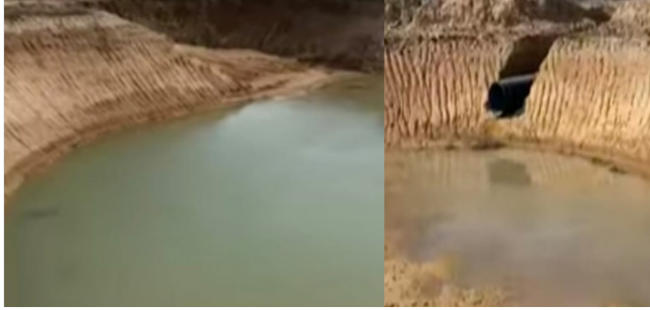
Kırklareli Water Storage Pool
